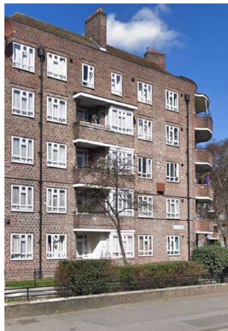
04 phase 6 stacked balconies
