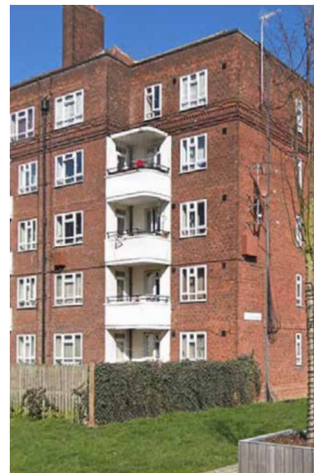
05 phase 4 corner balconies
